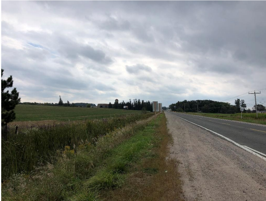
Plate 2: Yonge Street, looking south from Southview Avenue with active agricultural fields on both sides of the roadway (A.S.I., 2021).
