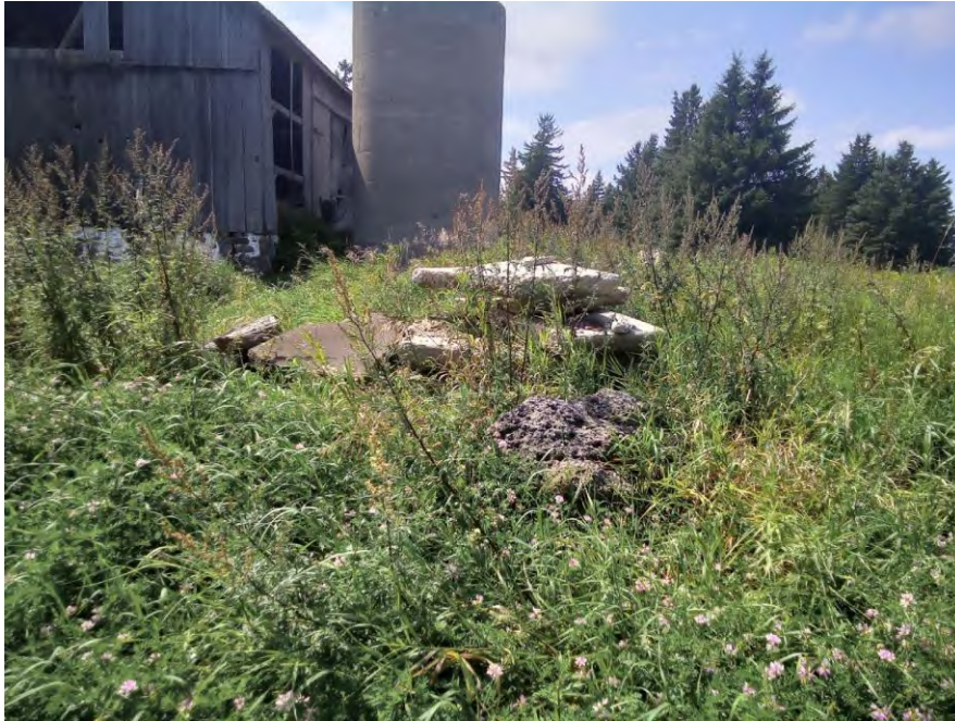
Image 11: View of demolished structure within the farm complex (2023).
