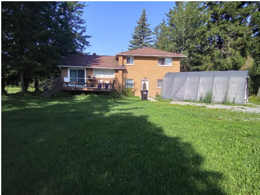
Image 2: View of the back of the house in the west of the subject property (2023)
