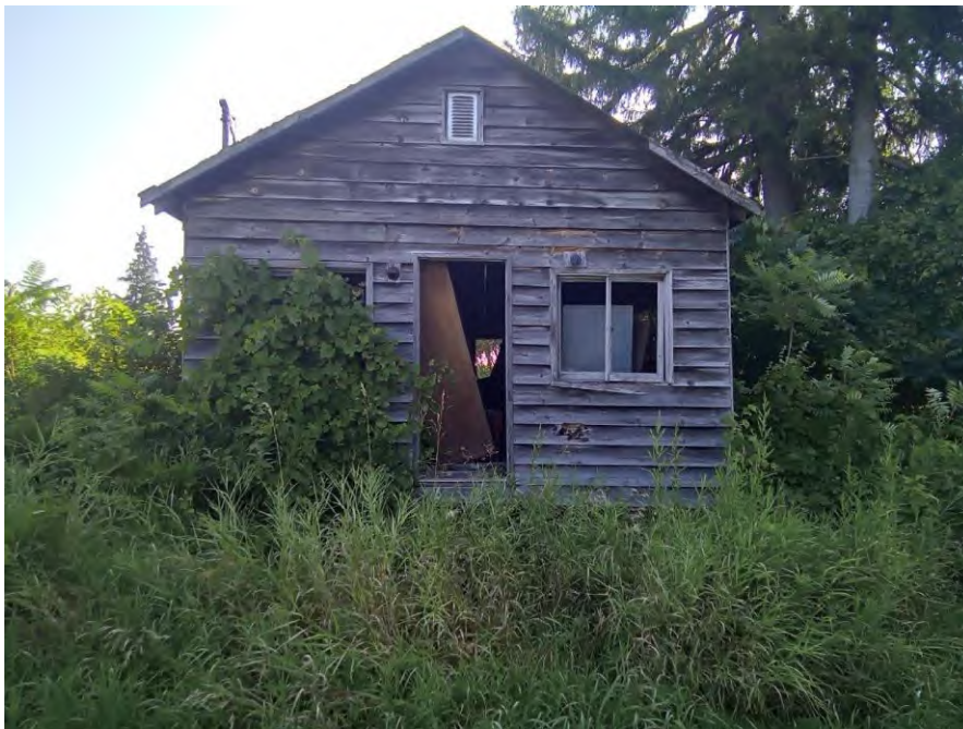
Image 10: View of an outbuilding within the north part of the farm complex (2023).
